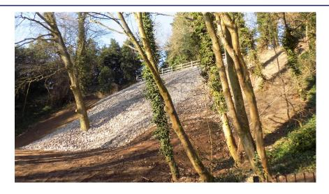
This contract was undertaken to remediate a landslip which had occurred to a steep river escarpment slope at Shrewsbury School, Shrewsbury. The steep, vegetated embankment within the ownership of the School failed following heavy rain in June 2018 when a section of retaining wall collapsed precipitating the landslip. The collapse caused damage to the adjacent Ridgemount Lane, damaged existing services and felled a number of mature trees growing on the slope.
